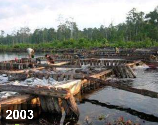
dams built by local communities with traditional techniques
